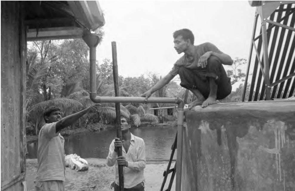
Figure 3.4: Fittings of interconnection pipes and funnels to guide water from gutter into the storage tank.
