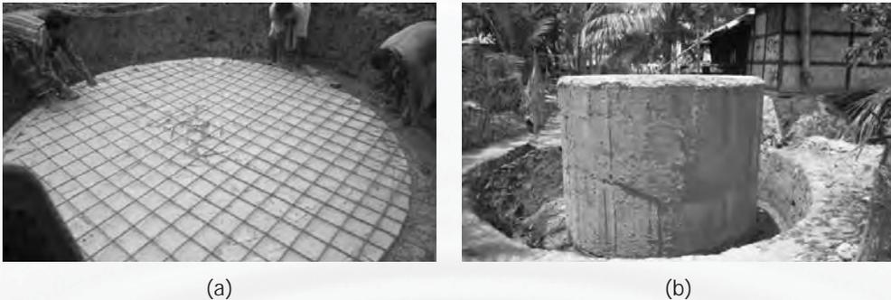
Figure 3.3: (a) Reinforcement for base of the storage tank
