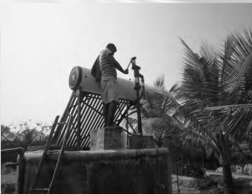
Figure 3.8: Lifting water into solar water heater reservoir from storage tank.
